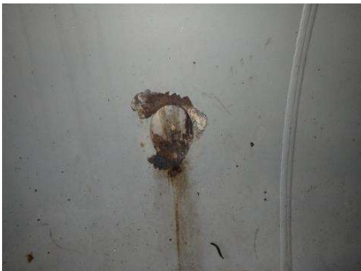
Typical Coating Failure around Nozzles
