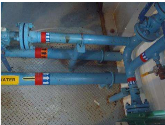
Produced Water / Sour Crude Outlet Piping
