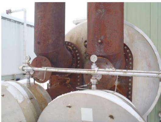
Fire Tubes and Stack
