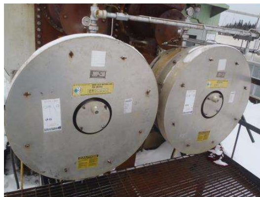
Spark Arrestors and Fuel Gas Piping
